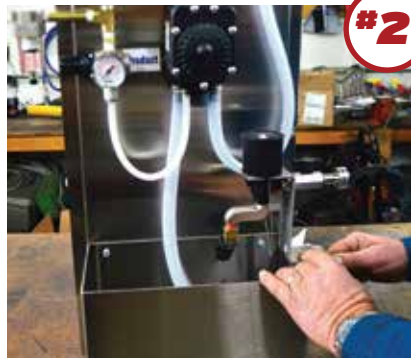
Mount the unit onto the wall in your control room. Next attach the provided Hydrominder to the side of the holding tank. Insert the tip of your choice depending on the chemical you use.
