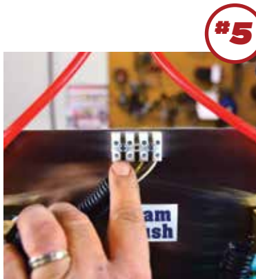
Next, run control wire for the foamy brush and the neutral from the coin box in your wash bay. Connect them to appropriate hook ups on the terminal strip on the top of the unit.
